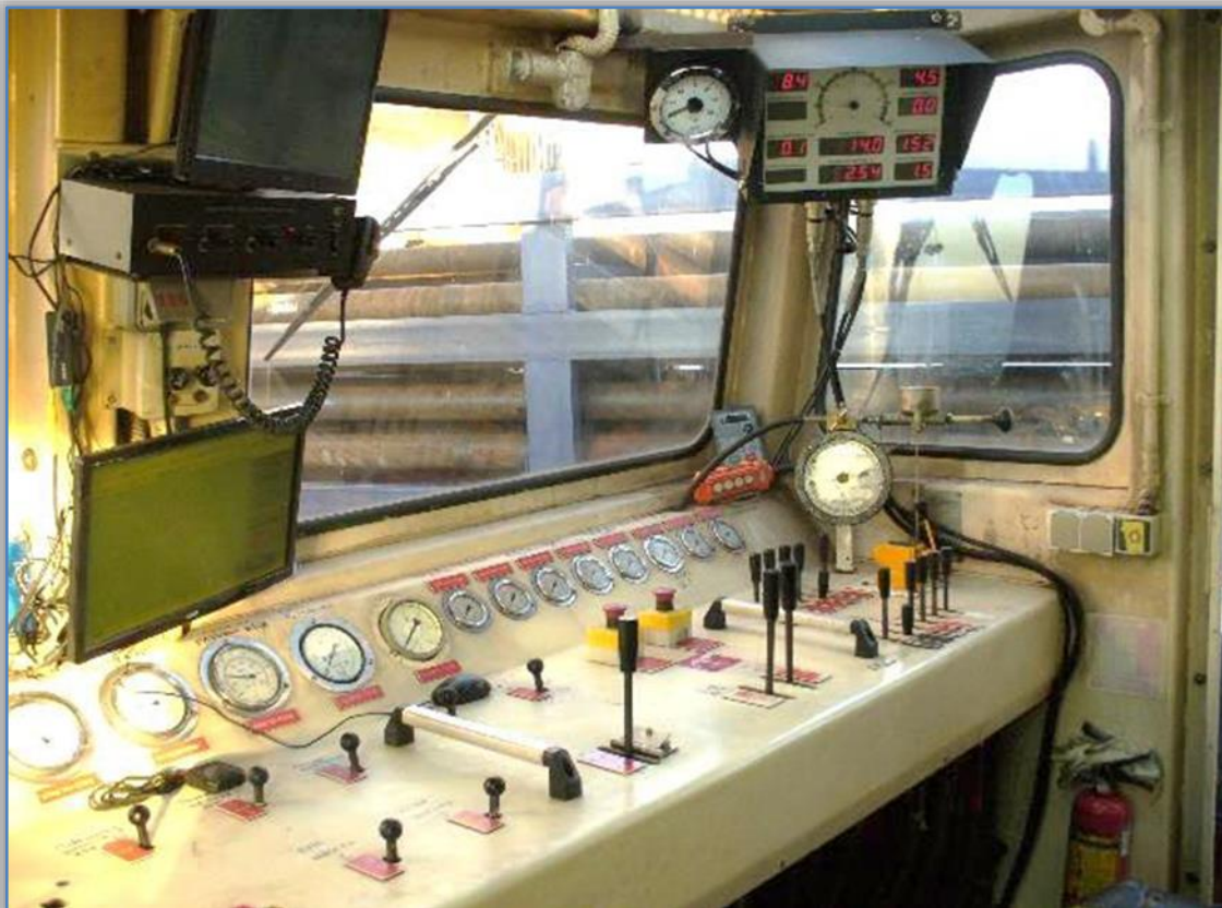
Drilling Rig Control Panel
