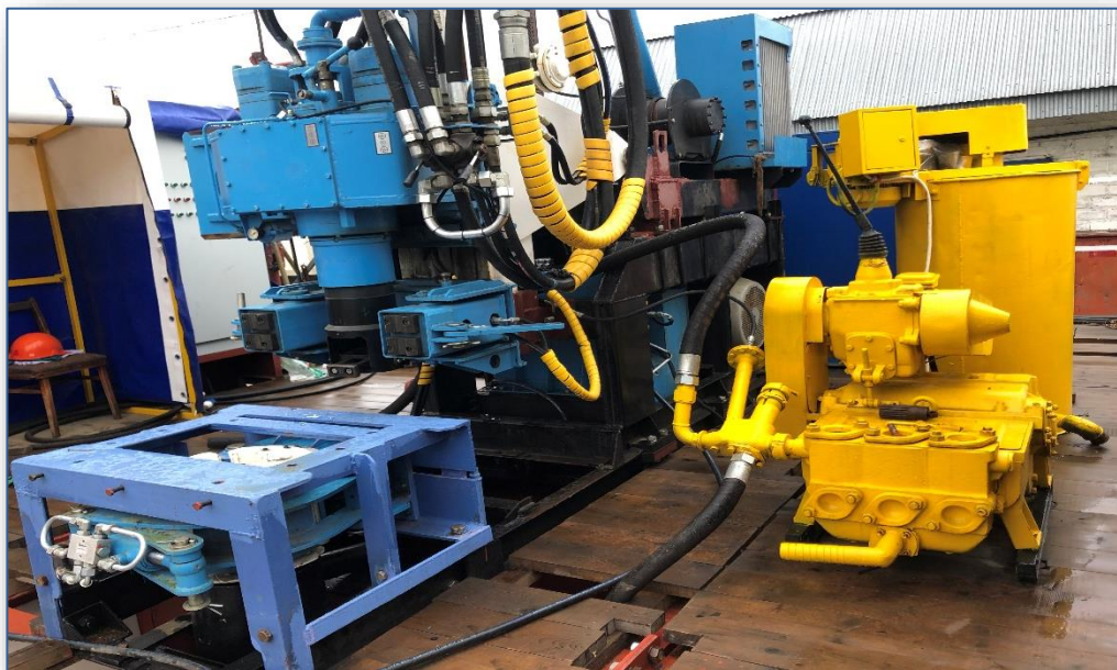
Power swivel of Drilling Rig. Mud pump NB-4
