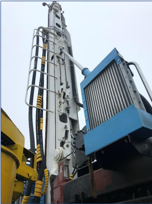
Drilling rig URB-41
